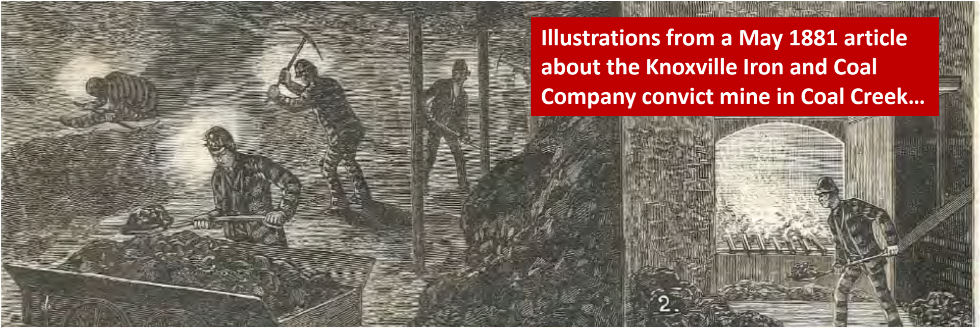
1. Within the Mine. 2. The Ventilating Furnace. 3. Loading Cars by the Chute. 4. The Entrance to the Mine.
